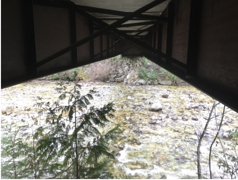
Left Bank Abutment when facing downstream
