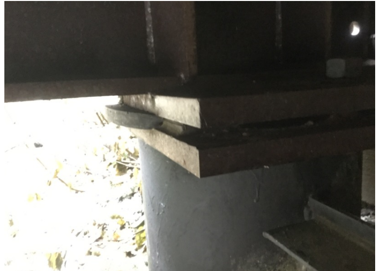
Upstream right bank bearing pads
