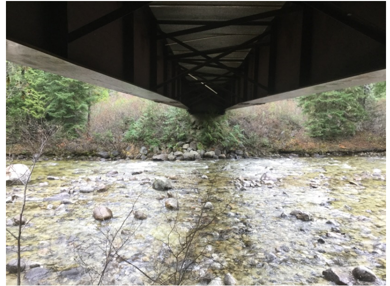
Right Bank Abutment when facing downstream
